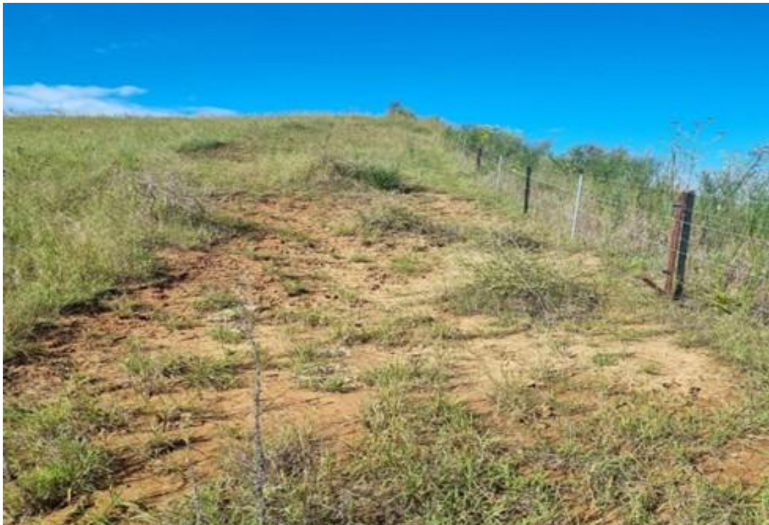
Photo 21 - Eroded ground above Medhurst Road batter
